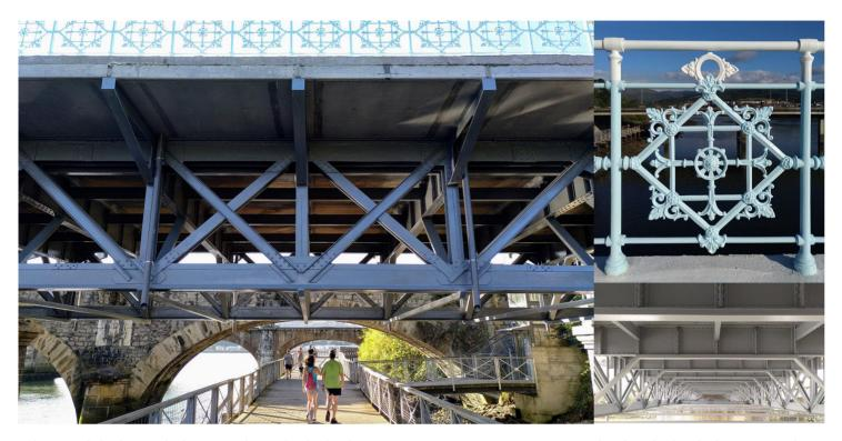
The Avenida bridge was built in 1915, being the third Bidasoa crossing in Irun after two masonry vault railway bridges built in 1864 and 1912. Between 1915 and 1966, it was the pedestrian and road link between Irun, Spain, and Hendaia, France. However, since 1966, this 112 m long truss bridge with five 22.40 m spans has been devoted to pedestrian use only.
